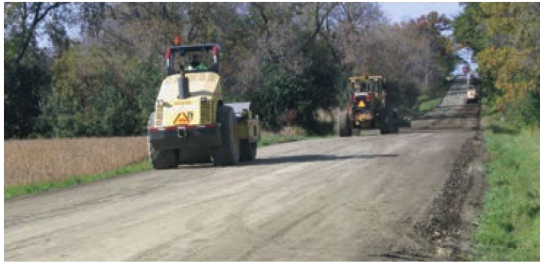
Fly ash-stabilized base being compacted on CTH BI in Dodge County.
